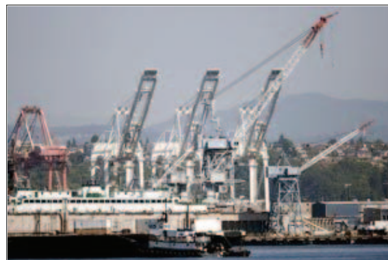
DANIEL HOUGHTON / THE SEATTLE TIMES Tenant SSA Marine took occupancy Monday at Terminal 30, two months later than planned because a trench was built too narrow for the cranes' electrical cable.
